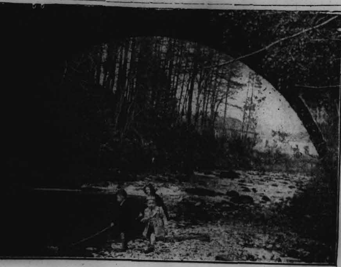
The Old Stone Bridge at Colligan.
