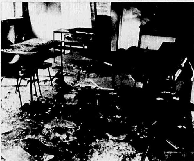
A burned out shell was all that was left of the former Deise Day Care Centre at Mitchell Street, Dungarvan after a serious arson attack. As a result of the fire, the smouldering wreck of the one-storey pre-fab building is thought to be structurally unsound and may have to be demolished.
