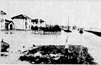
Clonea Road at Sallybrook which was badly flooded, with the high tide coming in over the sea wall.
