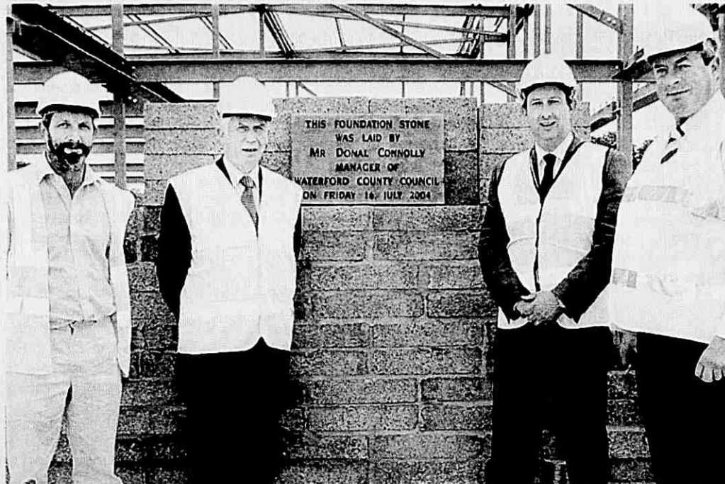
Laying of the Foundation Stone at the development of The Golden Meadows Retirement Village at the Burgery, Dungarvan were (left to right): Gerry Clancy, Clancy Construction, Donal Connolly, Co. Manager, David Reynolds, Sherry Fitzgerald Reynolds and Danny Lordan, M.D. Golden Meadows Retirement Villages.
