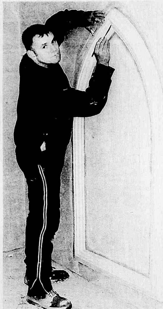
Well done to Timmy Coughlan from Cappoquin on getting 9 credits which earned him a merit, in his plastering apprenticeship and putting a finishing touch to his Gothic Arch.
