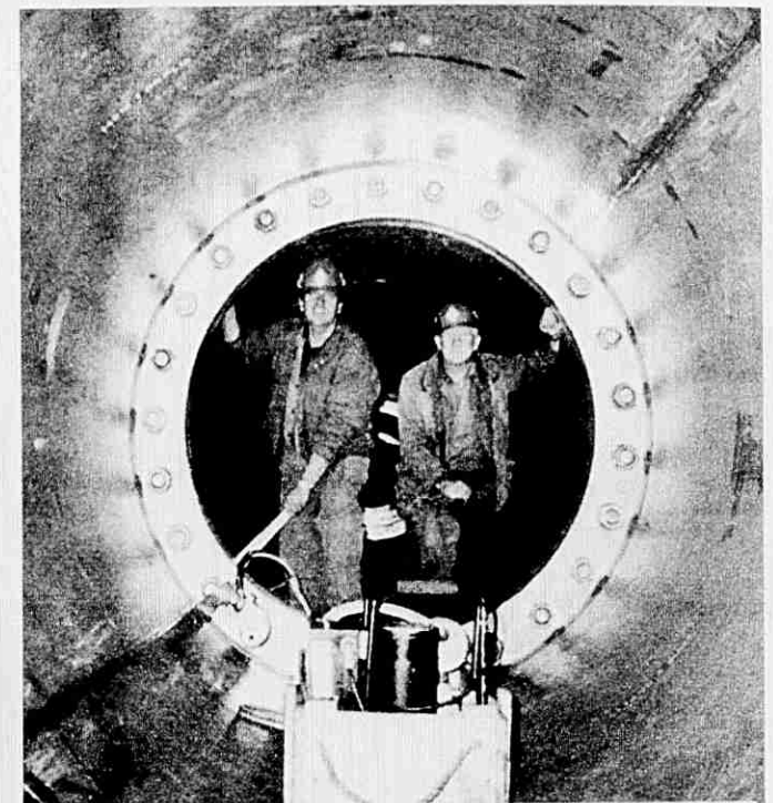
Pictures of the Millenium Spire being constructed at Radley's Enginnering Works in Dungarvan
