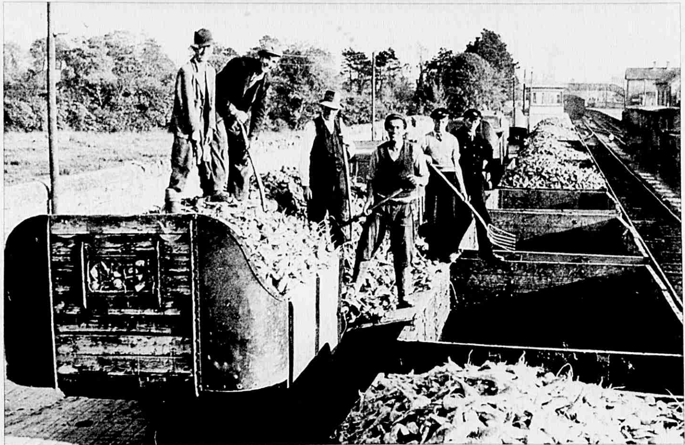
Working at the old Dungarvan Railway Station. From left to right: Matthew Hogan, Dick Curran, Dan Sullivan, Michael Flynn, Patrick Quirke, Patrick Croke. Photo kindly donated by Matthew Hogan. Anyone with any similar railway photos, please contact the museum on 058 45960
