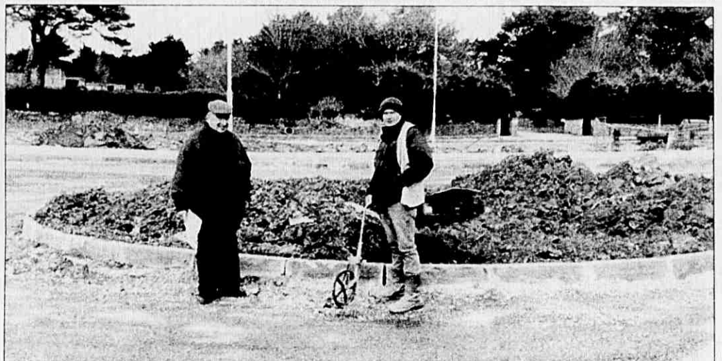
CLONEA ROAD ROUNDABOUT - Engineer Stan Connell and David O'Riordan with the trundle wheel take vital measurements at the almost completed roundabout opposite St. Augustines College at the junction of Boithrin a' Mhuilinn and Clonea Road.
