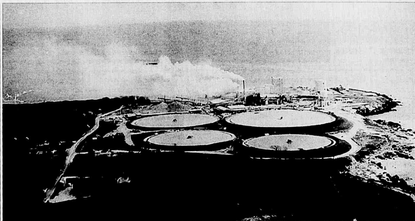
Full view of the Quigley Magnesite Plant at Ballinacourty with the big kilns in the foreground.
