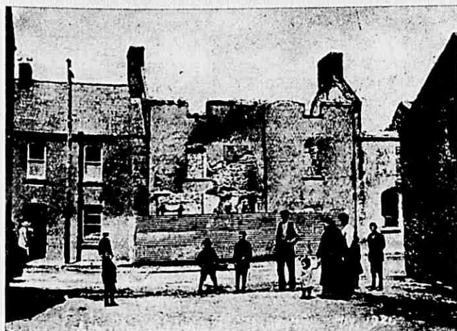
Mr. T. Fahey's House, Abbeyside (now Abbeyside Club) destroyed by fire. The houses to the right were also burned (Photo by Keohan).
