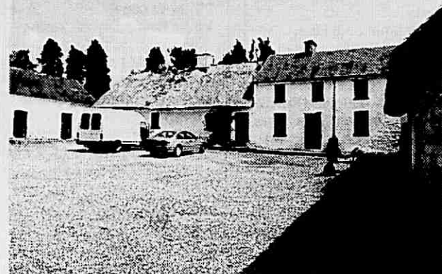
Delightful Thatched Farm House standing on its own. Renovations nearly completed.
