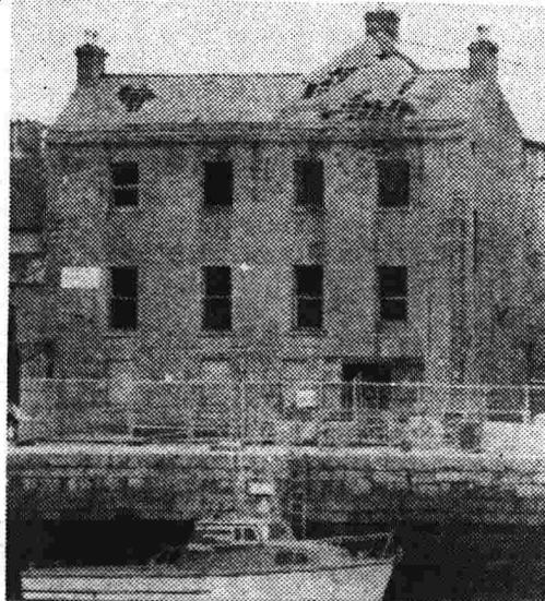
Impasse is resolved and work can go ahead on the old house and grain store on the Quay
