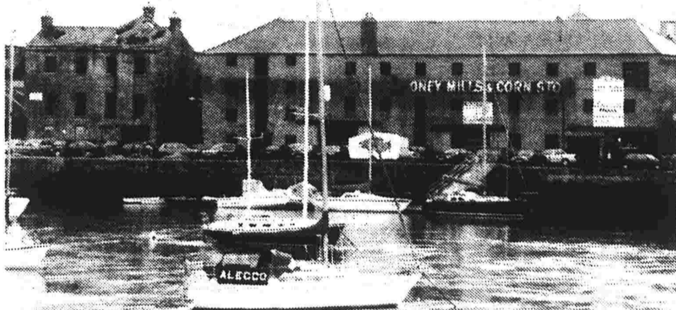
• Photo of the old Moloney Corn Stores building which was demolished to make way for a new four storey building by Clancy Construction.
