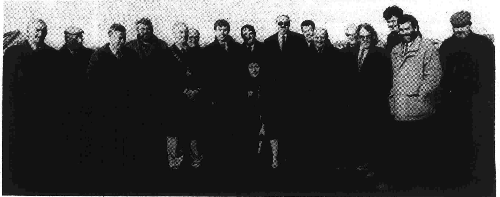
Cllr. Nuala Ryan, Cathaoirleach Dungarvan U.D.C. turning the first sod to mark the commencement of the construction of the Moray Properties Advance Factory at Clogherane, Dungarvan. Included are Ossie Spurling, Moray Properties, Cllr. Oliver Coffey, Chairman Waterford County Council, Donal Connolly, Waterford County Manager, Ray Moloney, Town Clerk, Muiris Críostóir, Architect and members of the U.D.C.
