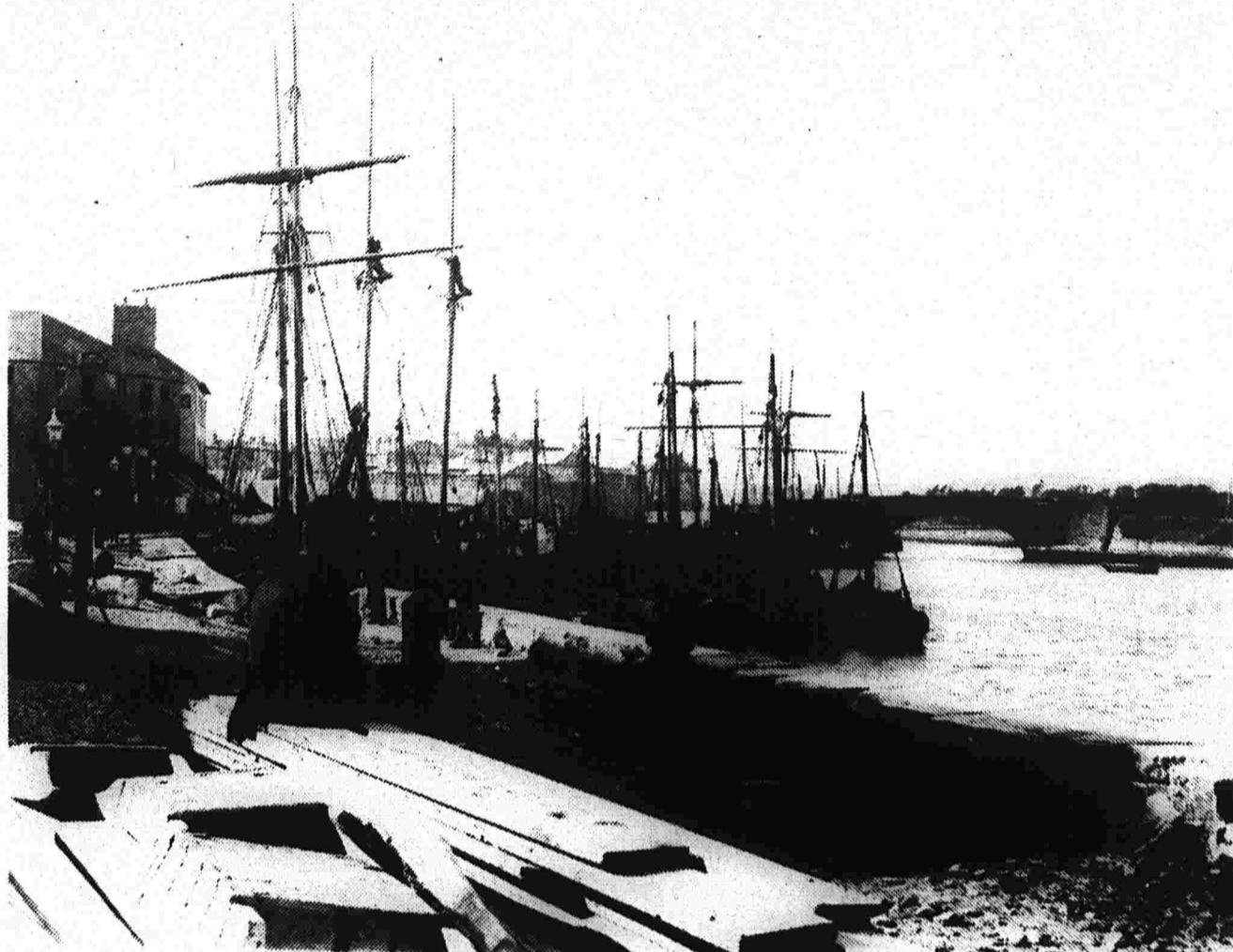
DAVITT'S QUAY — Under reconstruction in 1901. The Contractor was D. McGrath
