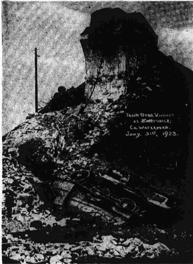
Train Wreckage At Ballyvoile (Photos by Keohan)
