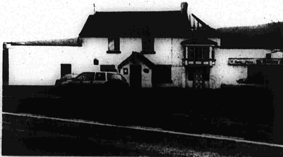
Hidden Inn, Kilmanahan, recently gutted by fire.
