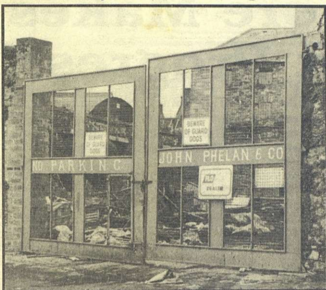
The shut gates at Phelan's Coalyard on the Quay as the site was being cleared last week.
