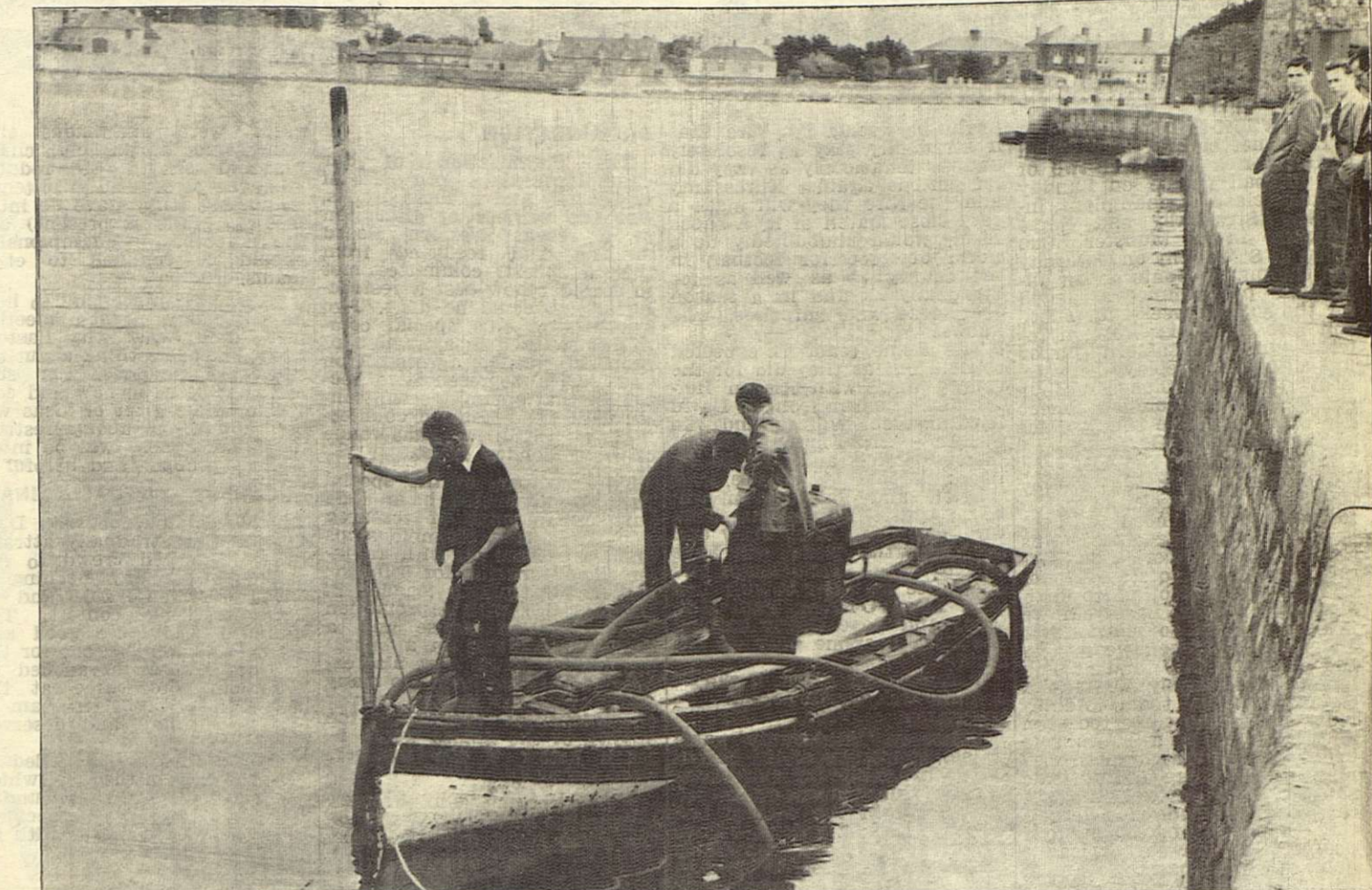
The photo for our "Remembering Other Days" this week is one taken from the Quayside in Dungarvan with Strands South, Abbeyside in the background. Taken by Tom Tobin in the early 1950's it shows Tom Kenneally, Convent Road in his boat from which the two men from the Board of Works in Dublin operated a suction pump in an effort to dislodge the mud-bank which was silting up the quay at the time. The operation was one sponsored by the Urban Council acting as the Harbour Authority but like other similar efforts to clear these mud banks, it proved a failure.
