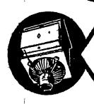
THE GRAIN DRIER is a fan and heater unit which will reduce the moisture content of grain safely and quickly. In practical operation it costs about 10s to dry one ton by 6%. There are three models evailable the 5KW size at £34 10 0 the 10KW size at £46 11 0 and the 15KW model at £65.5.0. These models will handle 300.600 and 1 000 barrels of grain respectively in a season
