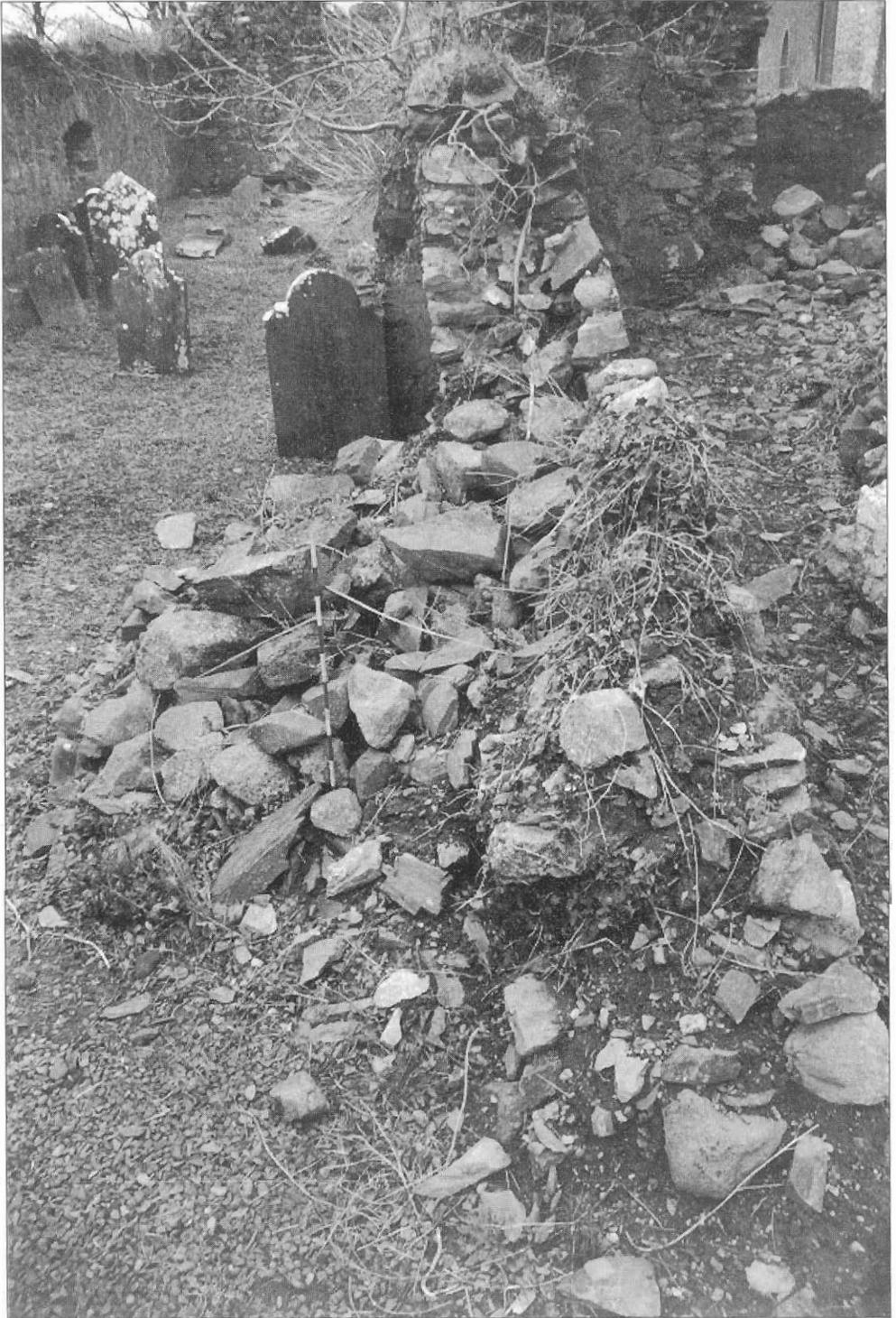
*Plate S – Collapsed clay-bonded section of north wall of chancel from east.*
