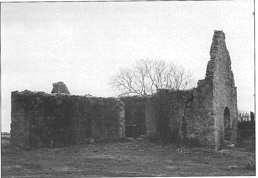
Plate 1: North wall of the church.
