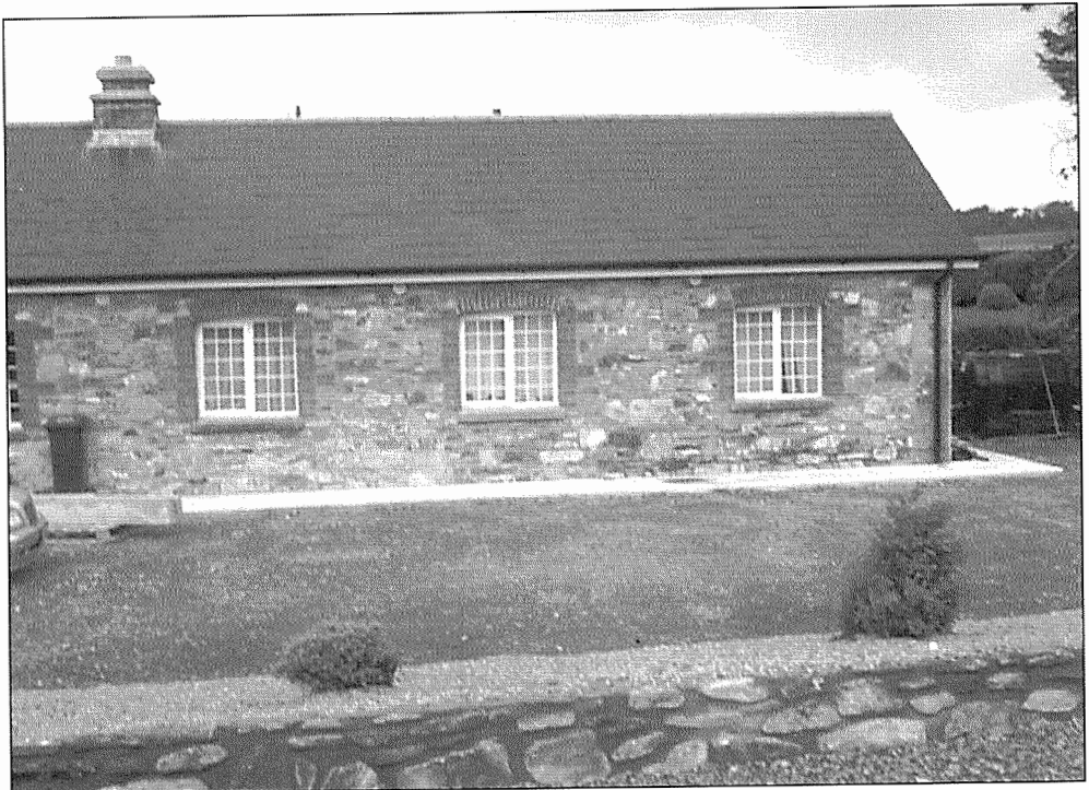
Plate 2: Renovated gate lodge.
