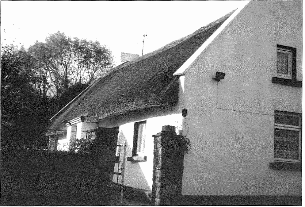
Plate 2: East facing gable.
